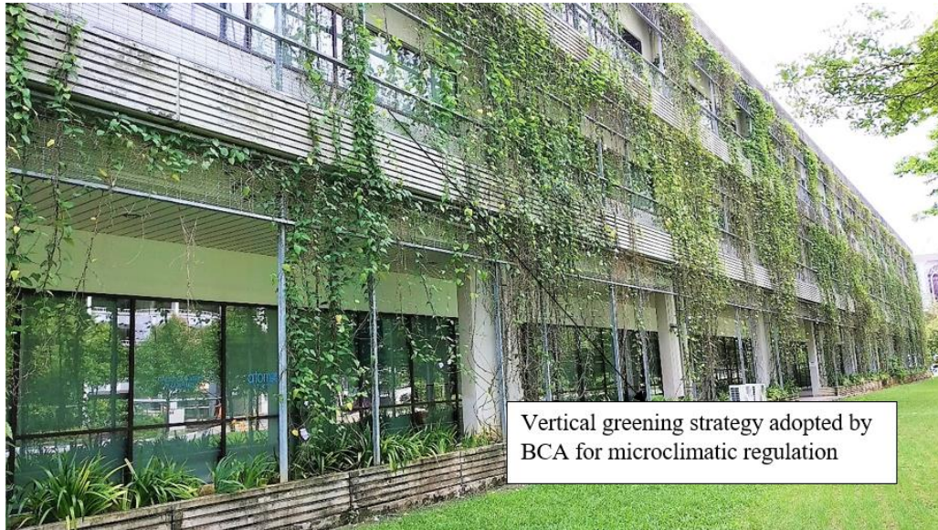
Image 5: Vertical Greening implemented by BCA at the site
